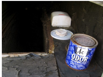
Several wall mounted aerosol deodorizers (left), and passive and aerosolized deodorizers placed within the roof top package units (right) were used in the facility. The facility spent approximately $1,100 annually on deodorizers in an attempt to “control” malodors.
